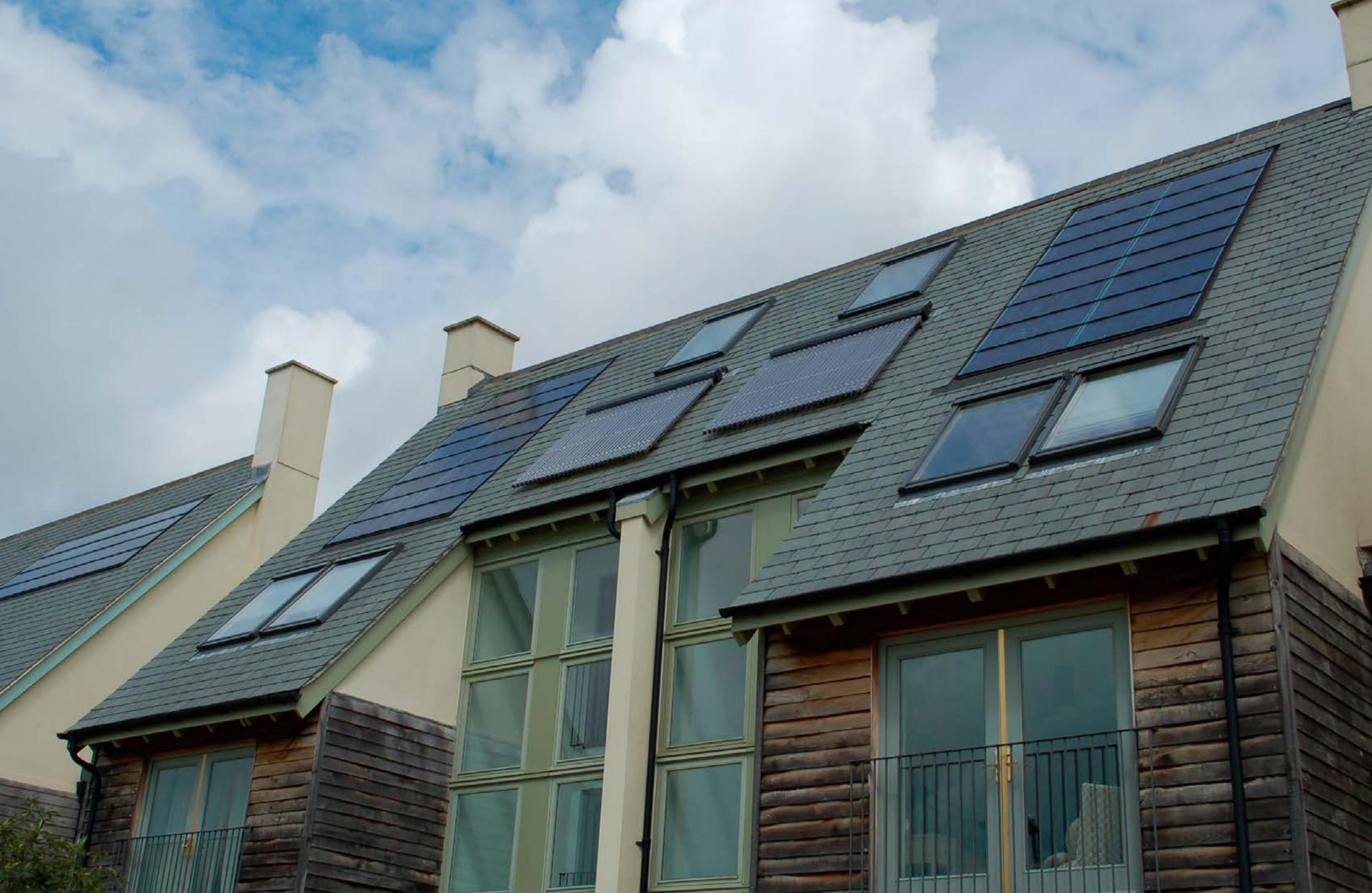
En3: Building orientation optimised for south facing roof area
