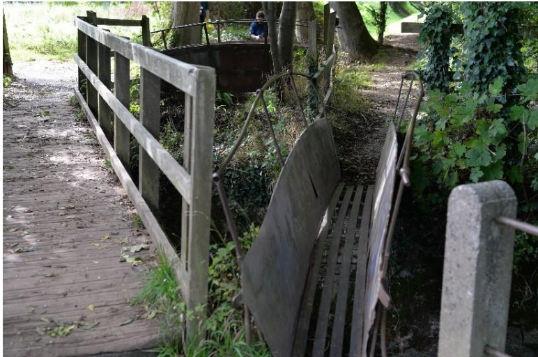
Photograph 10: Bridge crossing at the sump
