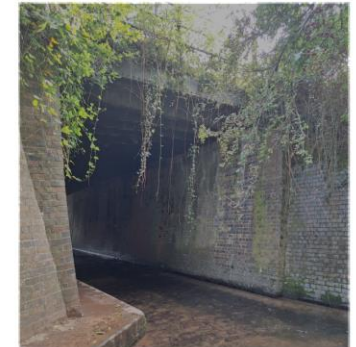
4 Railway bridge over the the Back Stream. The invert of this culvert is formed by cobbles embedded in concrete.
