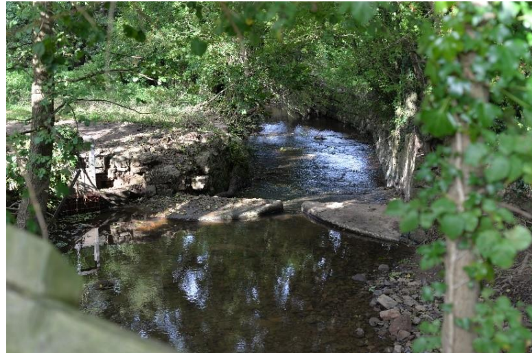
Photograph 13: Weir and sluice gate on Rockwell stream
