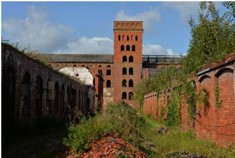
Figure 16. Tonedale Mill main building.
