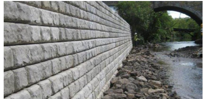
Figure 12. Examples of types of flood risk management options, (a) catchment scale management, (b) a leaky dam, as a form of natural flood management, (c) a flood wall, as a form of flood defence.
